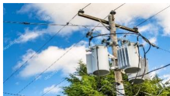
FIG.1.2:DISTRIBUTION SIDE TRANSFORMER
