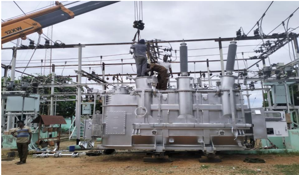
FIG.1.7:ERECTION OF NEW TRANSFORMER IN KOODALNAGAR EB SUBSTATION
