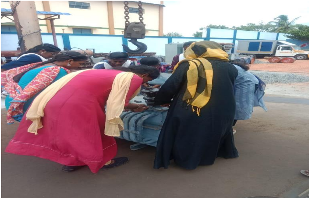
FIG 1.1 DISMANTELING THE TRANSFORMER
